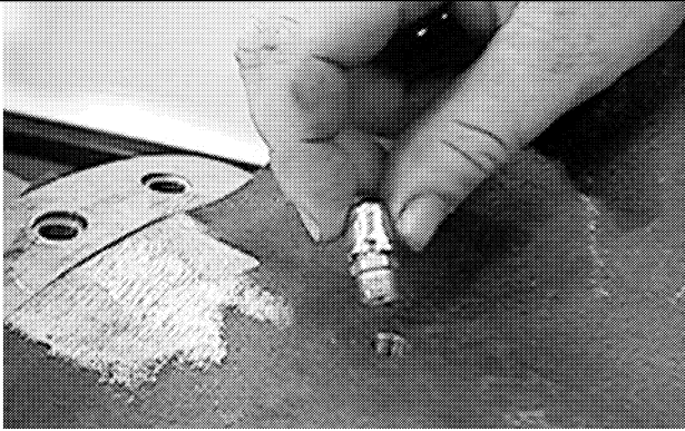
19j. Install vent in housing and torque to 7-10 ft/lbs. (9.5-13.5Nm)
