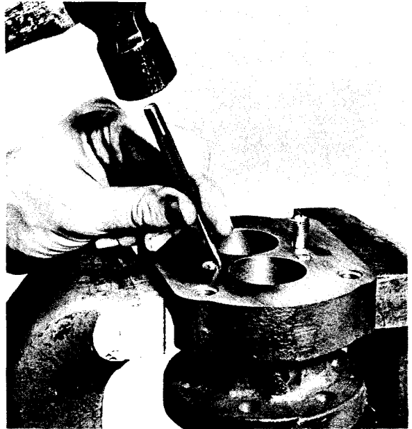
Fig. 5 Peening over check valve seat
